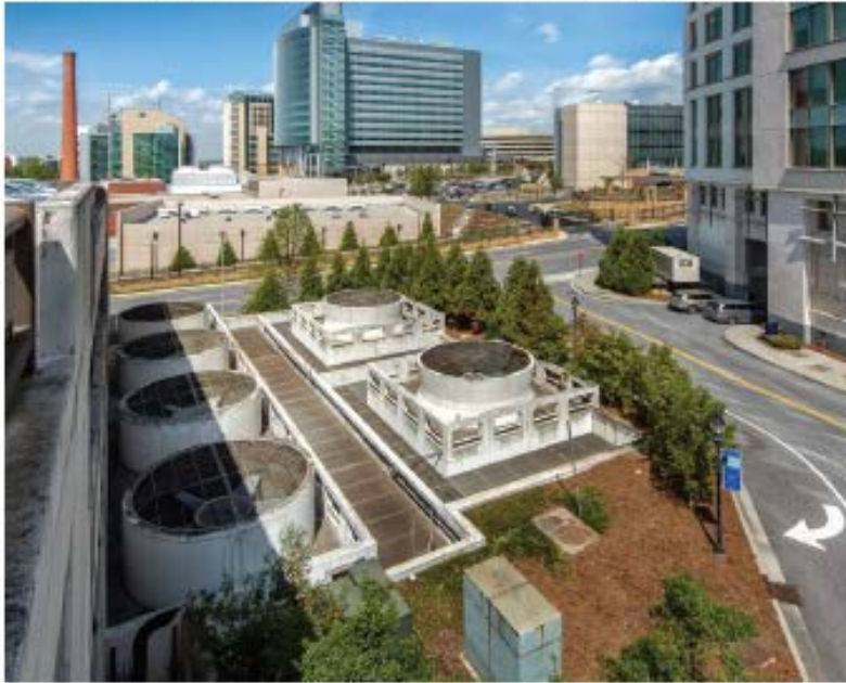
Cooling towers at Michael St. Chiller Plant now receive reclaimed water
