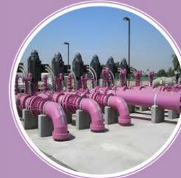
Recycled Water Supply & Distribution
