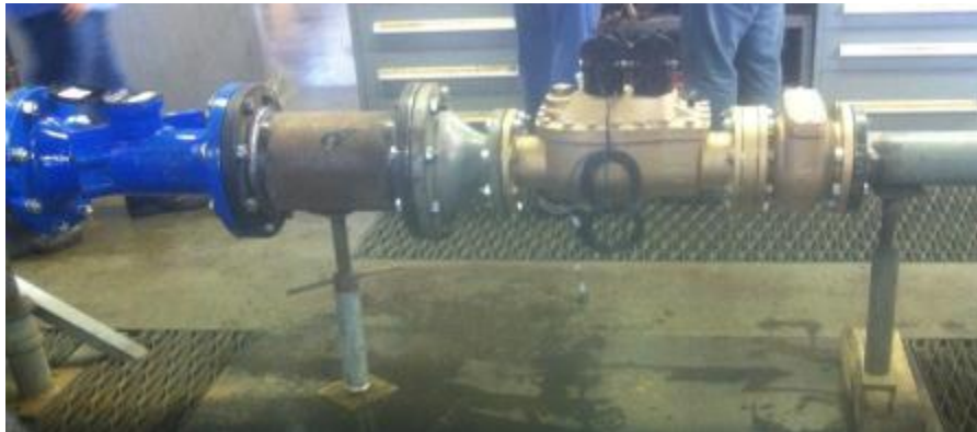
Ultrasonic meter installed on WV test bench
