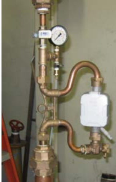
Ultrasonic meter for lower flow rates
