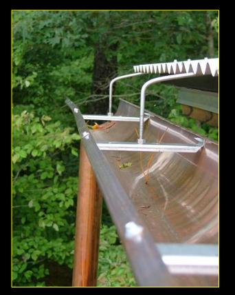
2 inch by 3 inch downspout = 600 square feet of roof top 600 X 0.623 = 374 gallons
