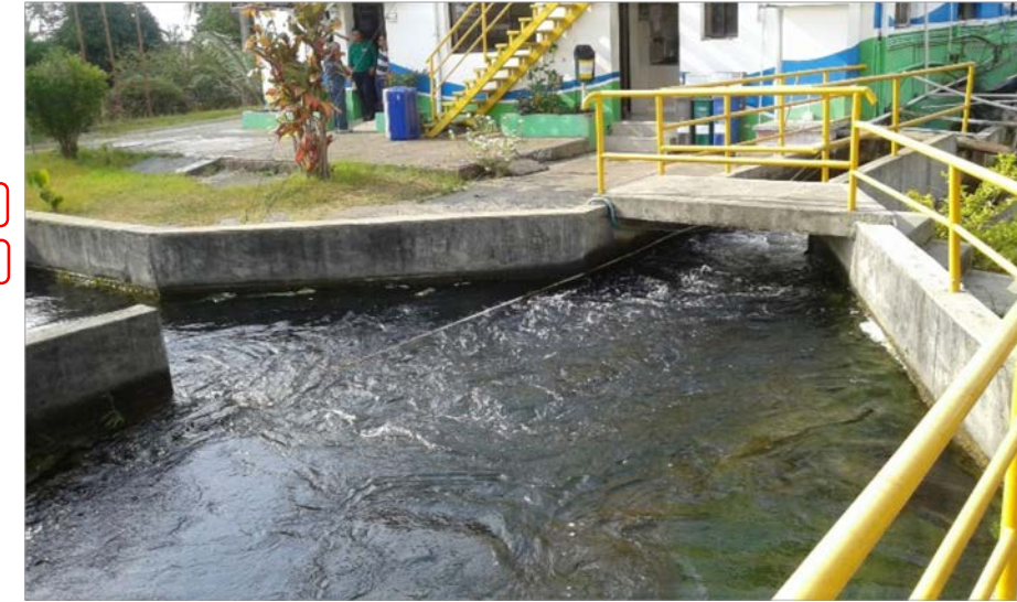
Municipal Drinking Water Treatment Plant Armenia (Quindío)
