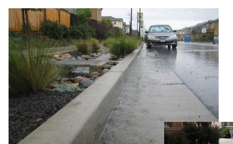
Bioretention treats storm water with soil and plant-based filtration
