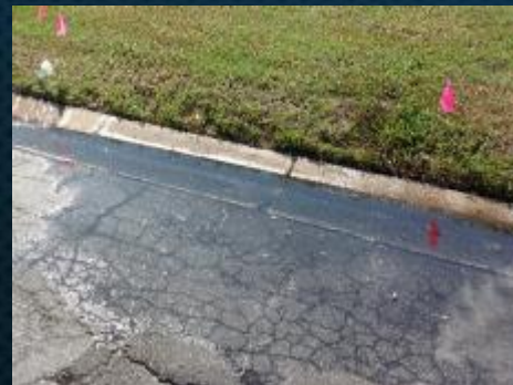
Damage due to broken lateral
