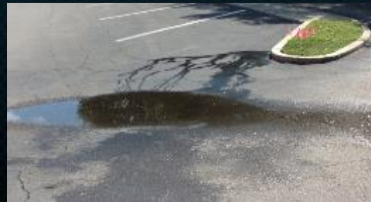
Hardscape Damage due to Runoff
