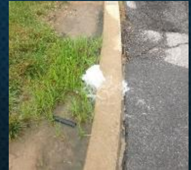
Landscape & Hardscape Damage
