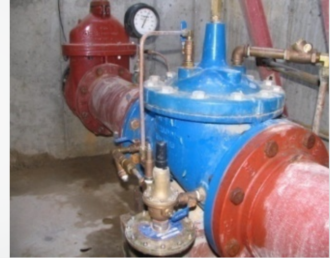
Pressure Reducing Valve used for pressure management installation in Philadelphia
