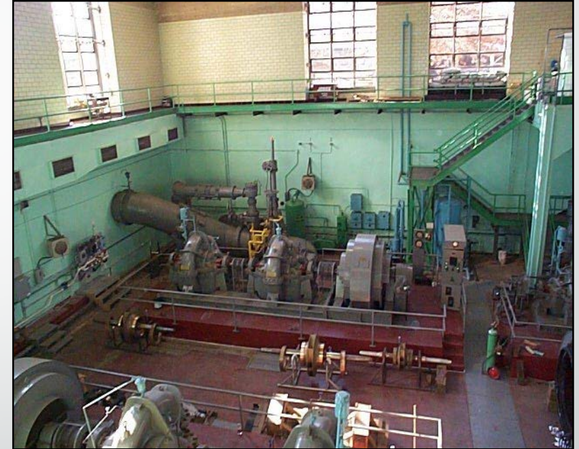
Queen Lane Pumping Station in Philadelphia
