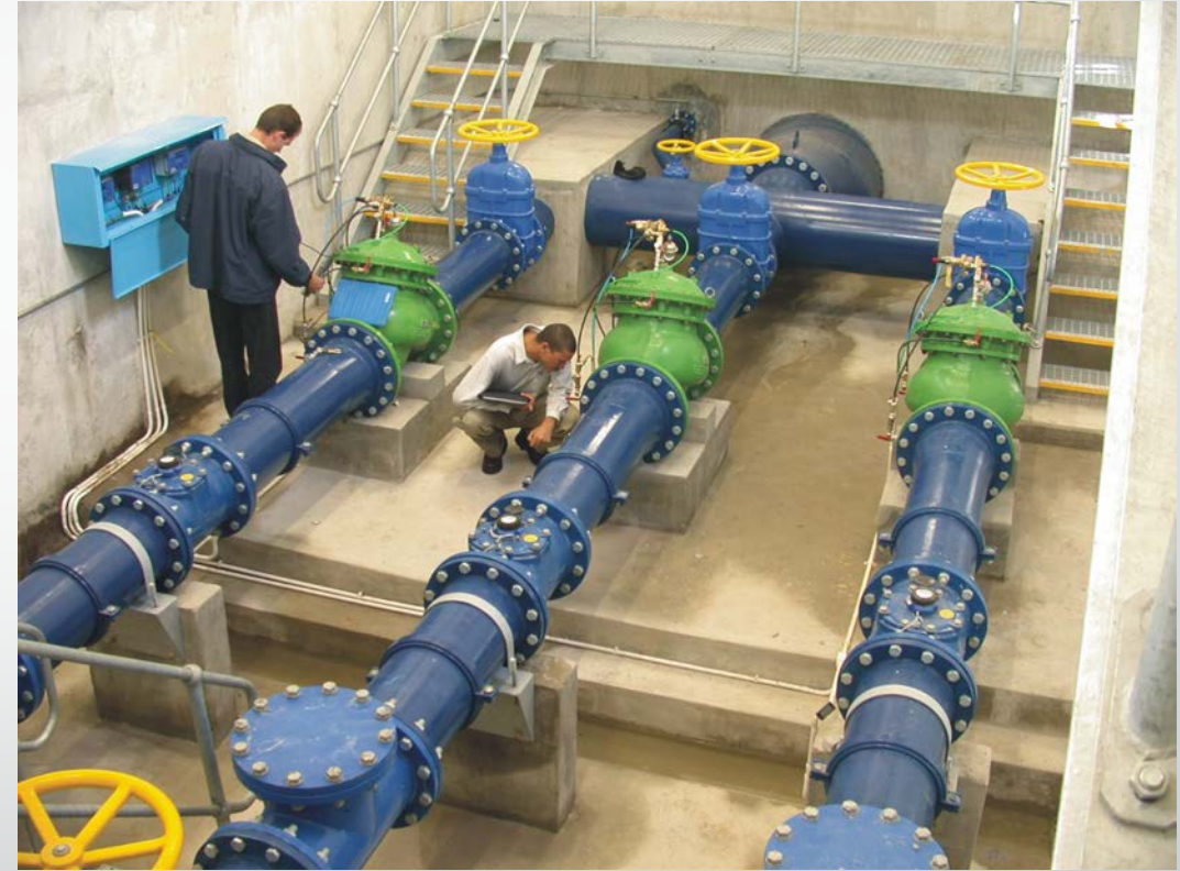
Large Pressure Management installation in South Africa Source: Ronnie McKenzie, WRP Pty Ltd.
