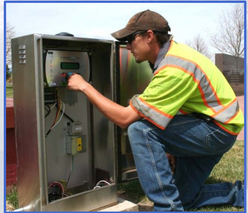
WeatherTRAK Controllers in use.
