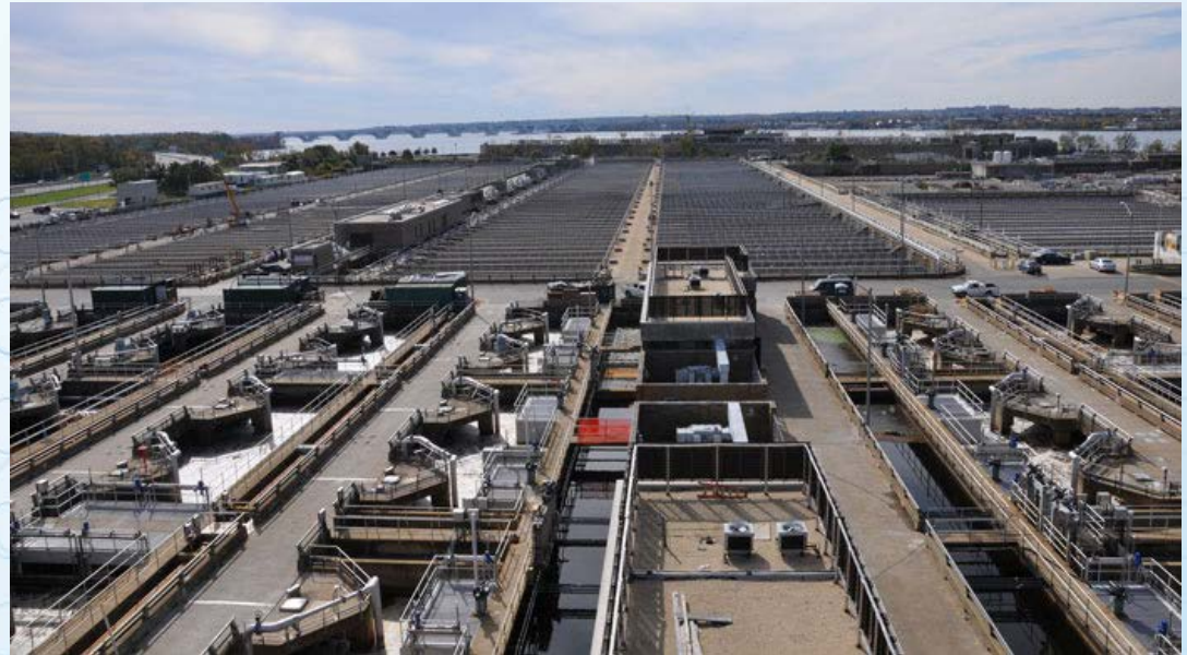
Blue Plains wastewater treatment plant
