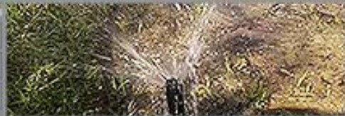
Damaged Sprinkler Heads
