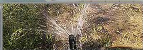
Damaged Sprinkler Heads
