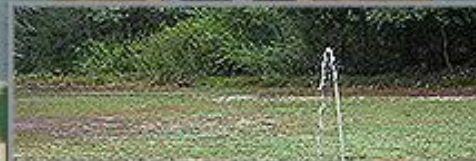
Clogged Nozzle or Filter
