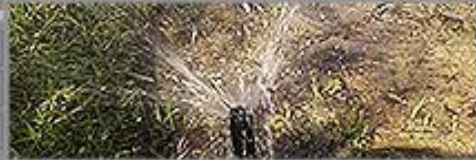
Damaged Sprinkler Heads
