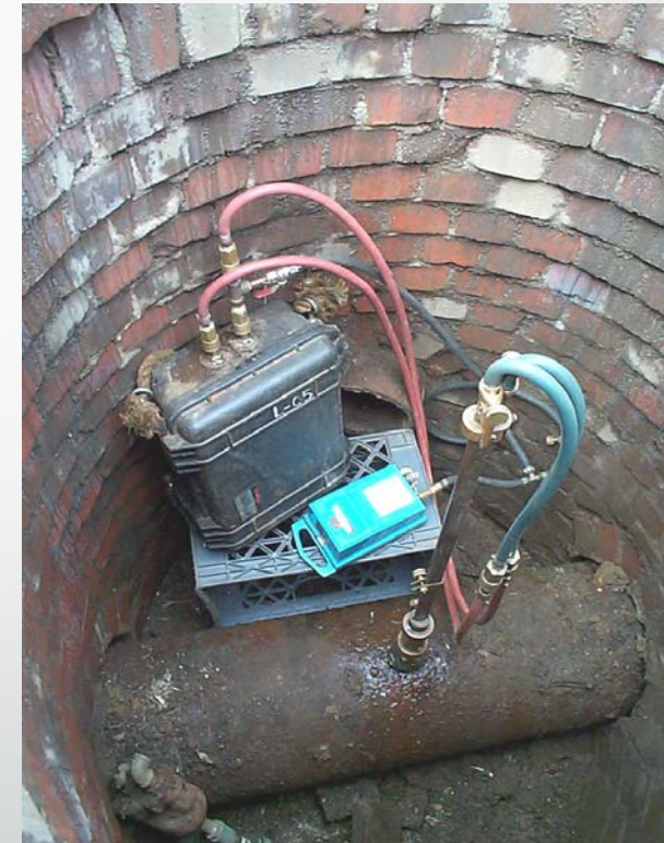
Insertion pitot rod measuring and recording flow
