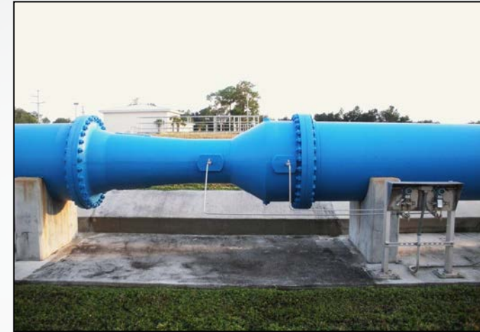
36-inch Venturi Meter (Courtesy of Primary Flow Control)
