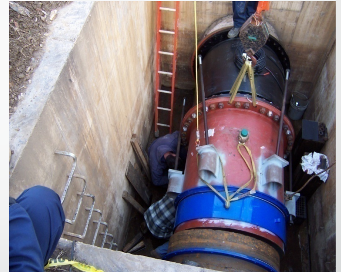
Magnetic Flow meter replacement on 48-inch untreated water line 2008 in Philadelphia
