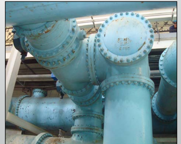
Maze of pipe bends downstream of above meter
