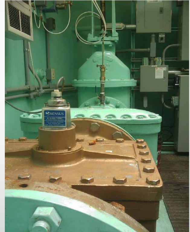
16-inch turbine meter on wholesale water supply pipeline being verified via inline pitot rod
