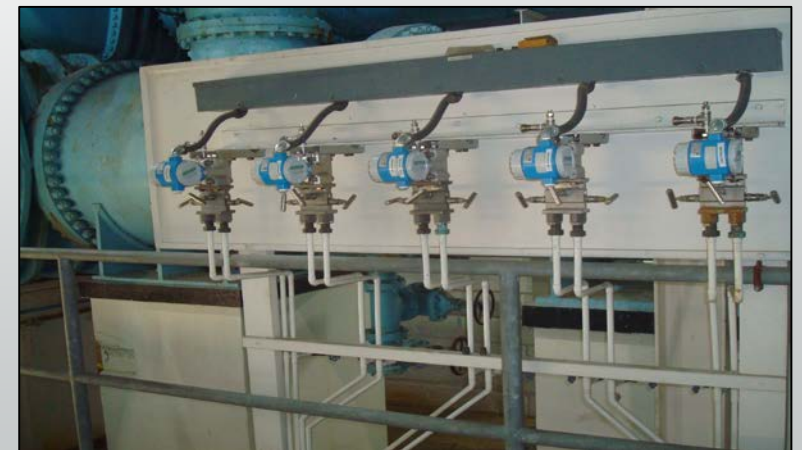
Bank of Differential Pressure Cells connected to flowmeters (Courtesy of Louisville Water Company)
