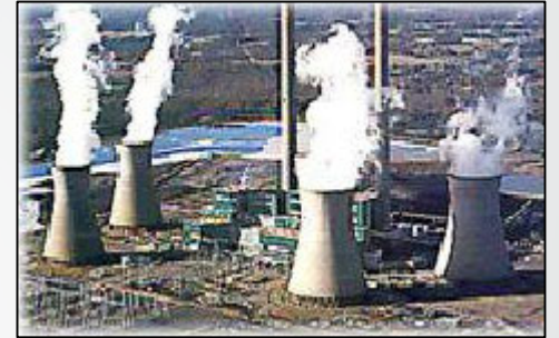
Thermoelectric Power 161 bgd Photo source: USGS
