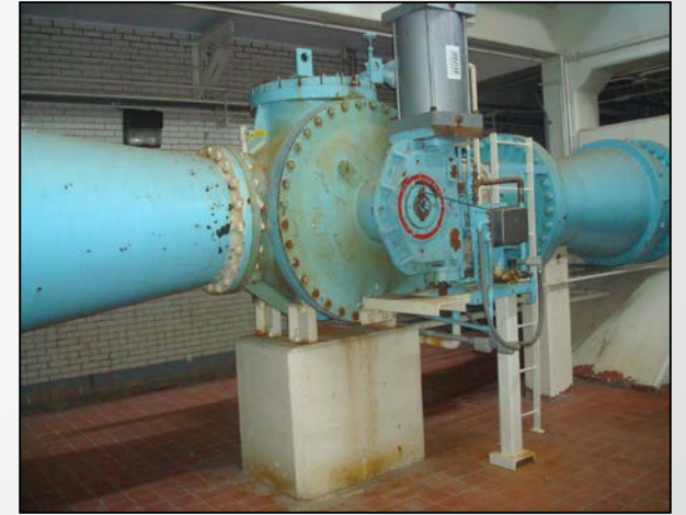
Venturi meter with valve in the throat
