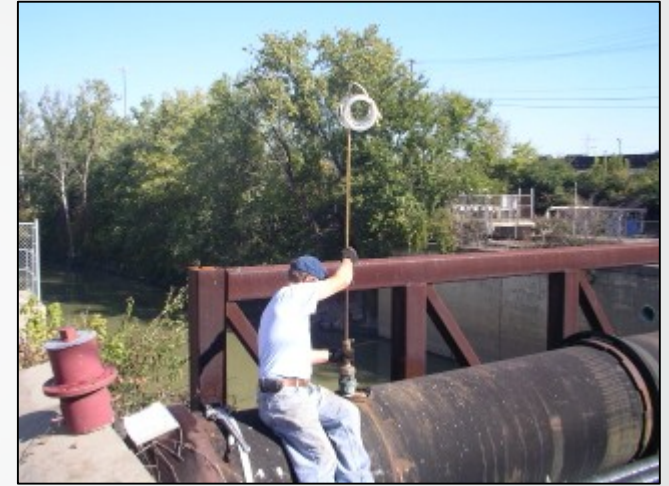
Pitot rod inserted into large pipeline
