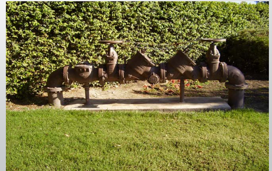
Poor meter configuration that doesn't allow testing
