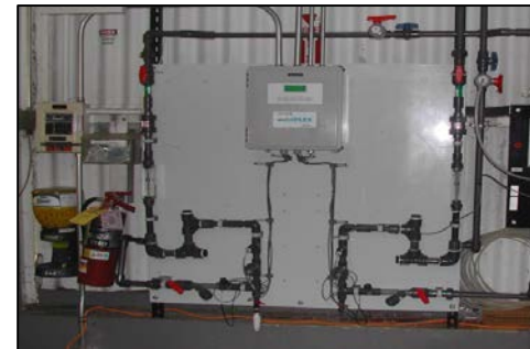
Advanced cooling tower controls
