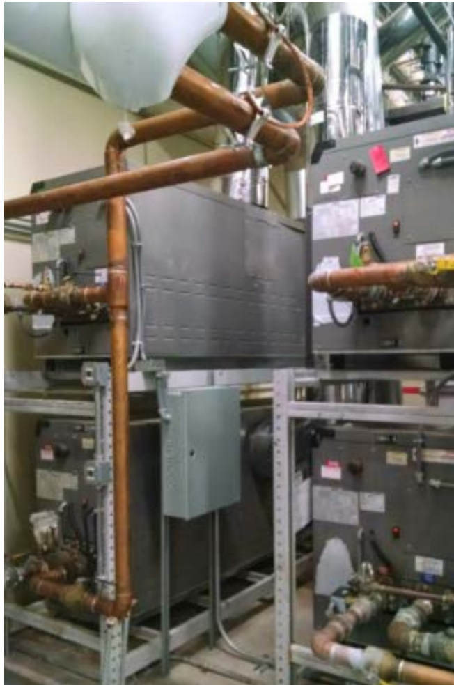
Boiler / Water heater
