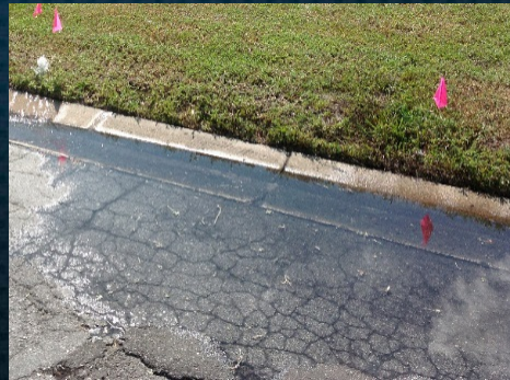
Damage due to broken lateral
