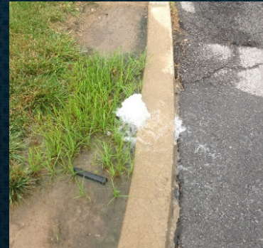
Landscape & Hardscape Damage
