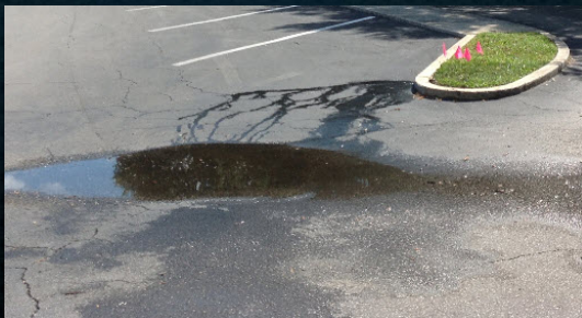
Hardscape Damage due to Runoff
