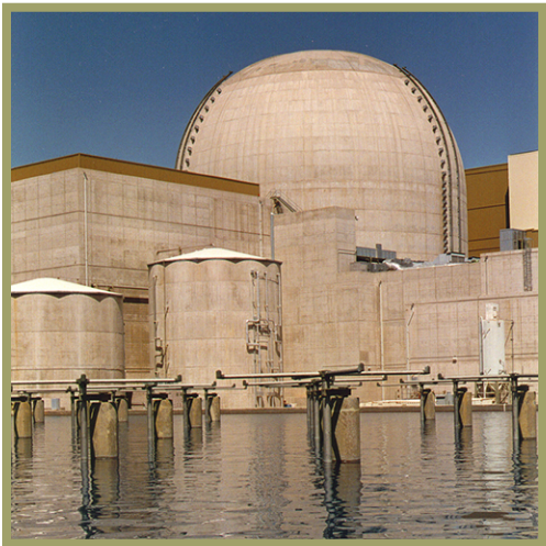
Palo Verde Nuclear Generating Station Photo: APS
