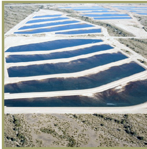
Tonopah Desert Recharge Project Photo: City of Glendale
