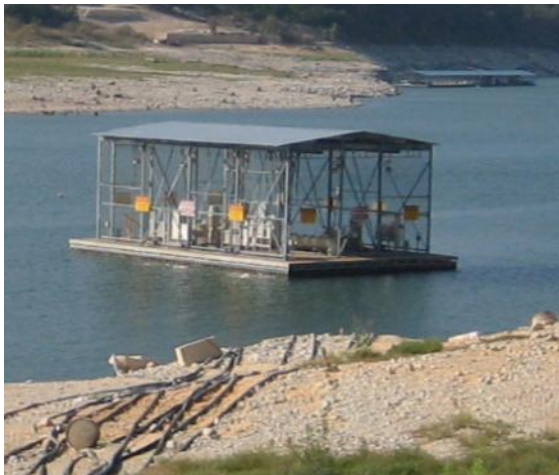
Floating Owned Pump Station
