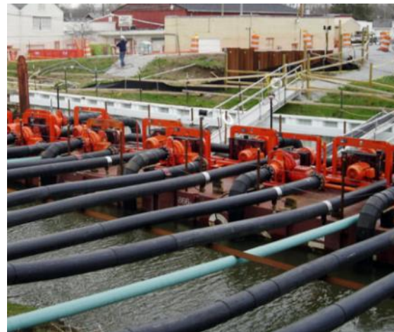
Floating Rental Pump Station
