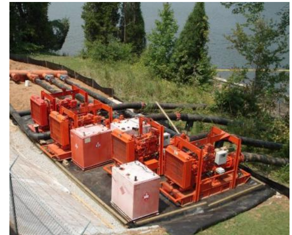
Land Based Rental Pump Station
