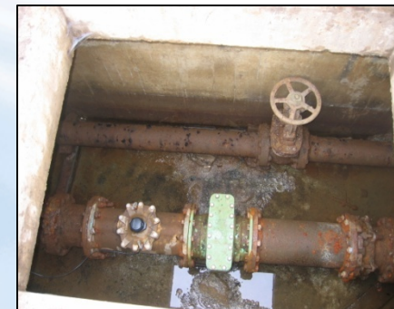
10-inch Badger Turbine Meter at medical facility
