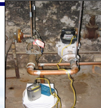
10-inch Badger Turbine Meter at medical facility
