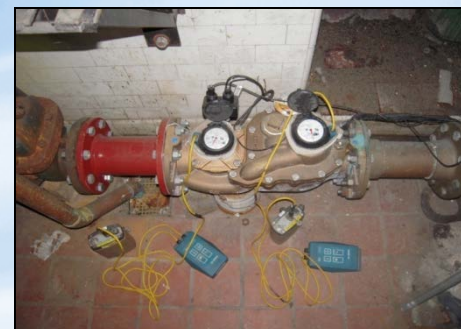
10-inch Badger Turbine Meter at medical facility
