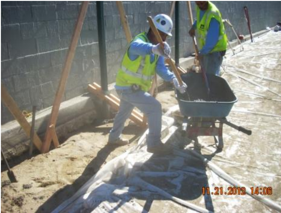
Concrete for green screen footings.
