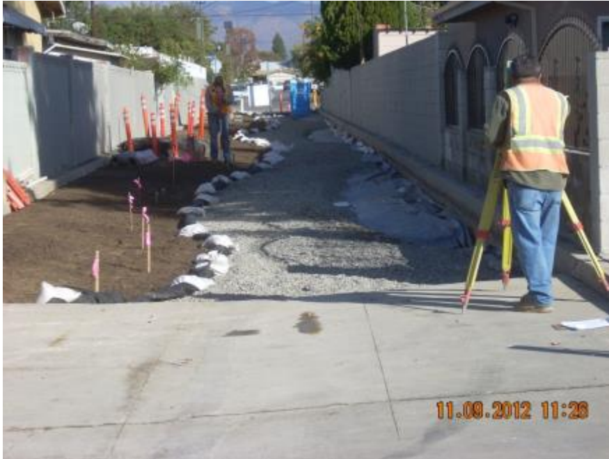
Survey for pathway elevation points
