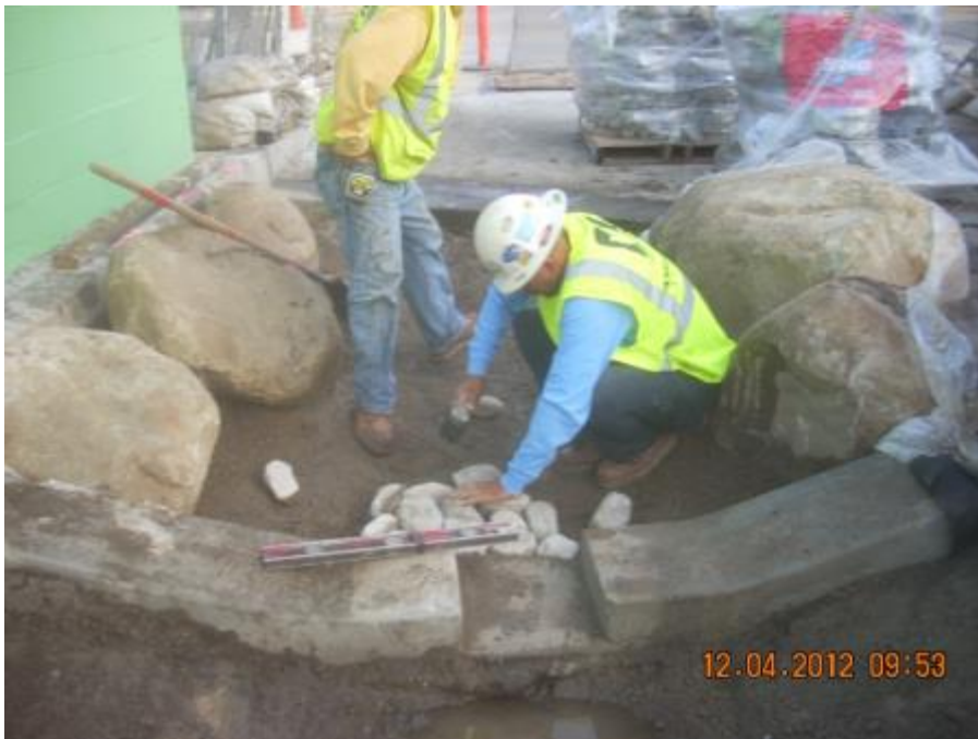
River rock cobble for bio-swale forebay.
