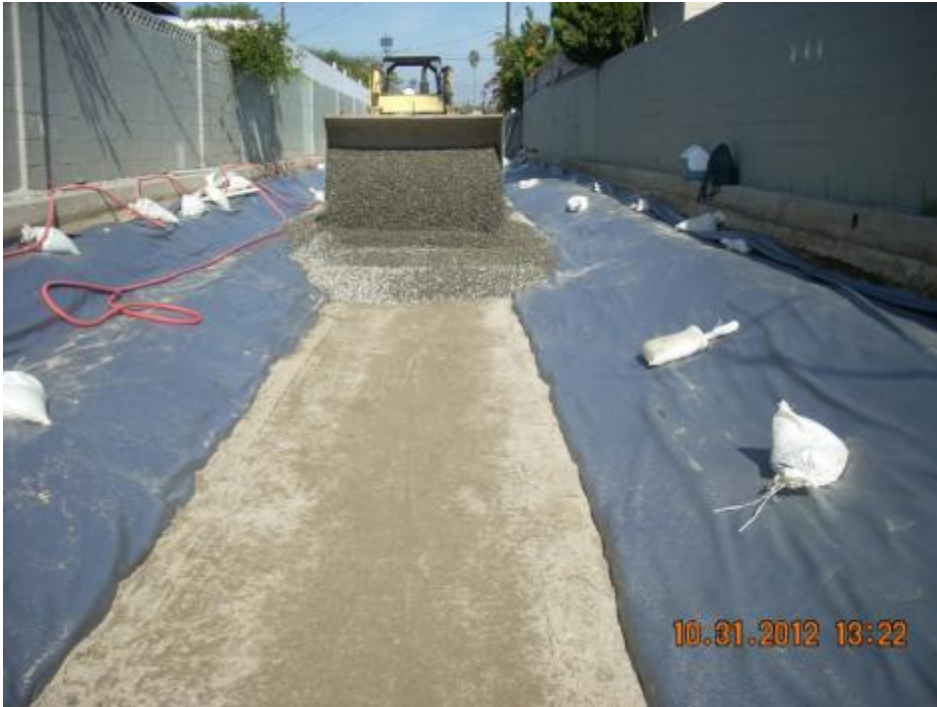
Installation of infiltration trench gravel
