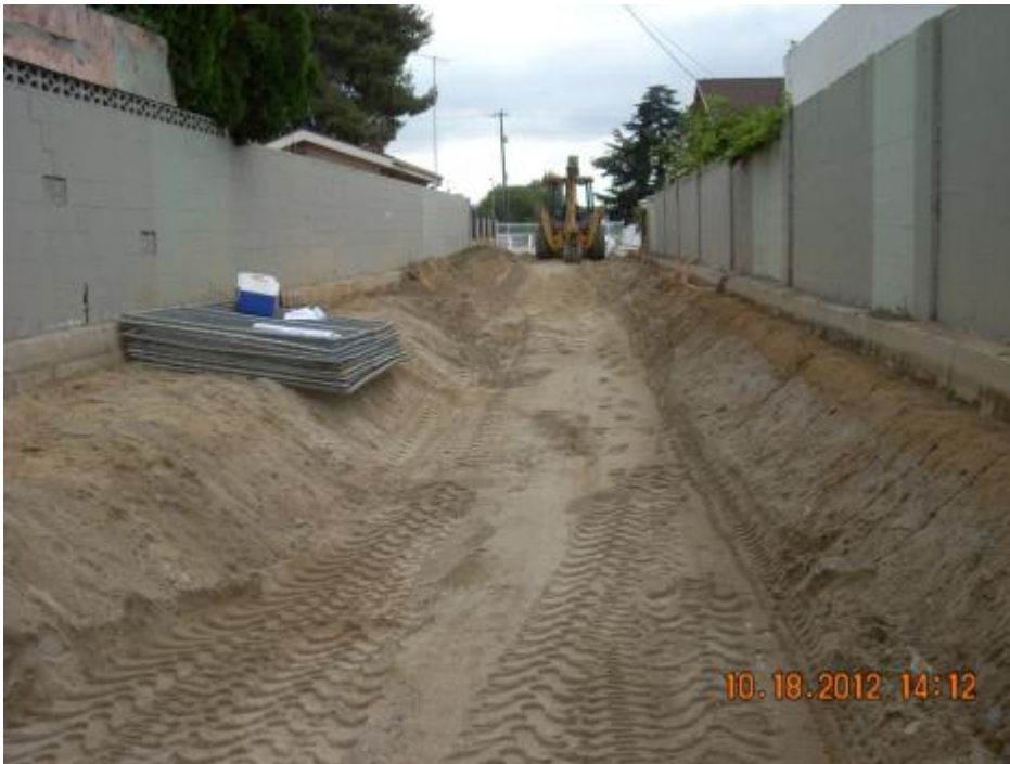
Excavation of infiltration trench
