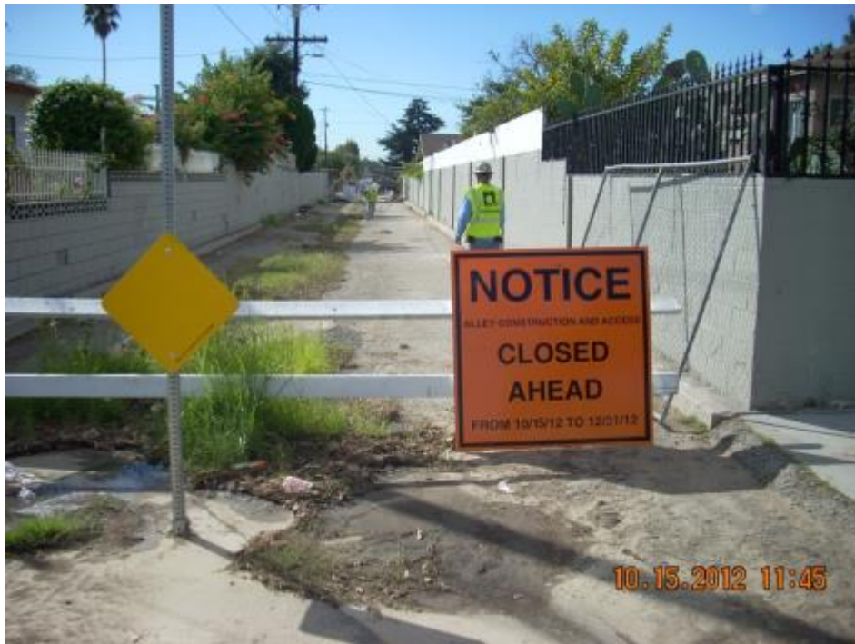
Demolition and removal of asphalt pavement
