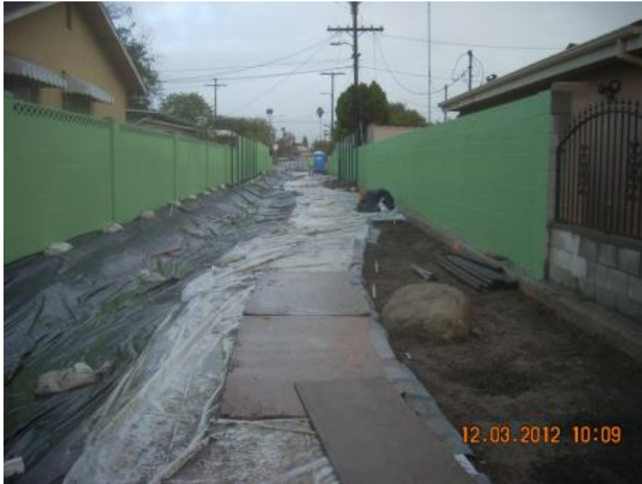
Letting the site dry out after rain.
