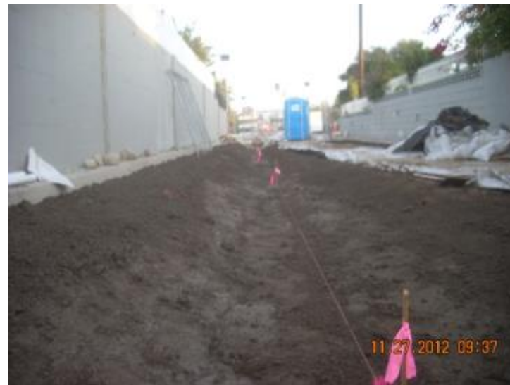
Elevation points set for bio-swale
