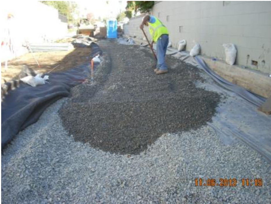
Construction of bio-swale, infiltration trench, and pathway continued.
