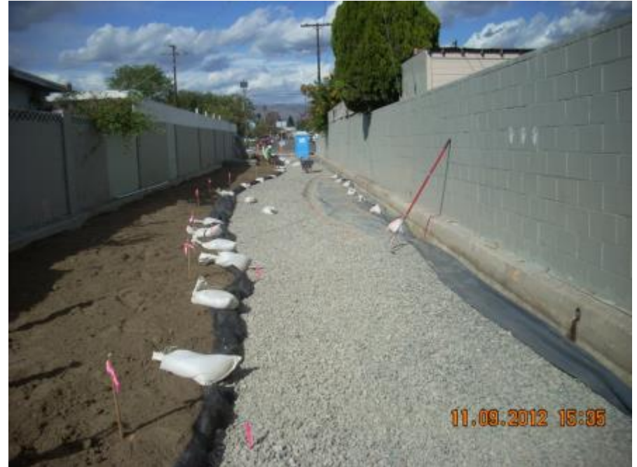
Base layer for pervious concrete pathway
