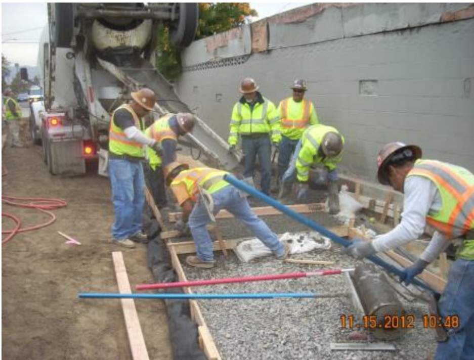
Construction of pervious concrete pathway.
