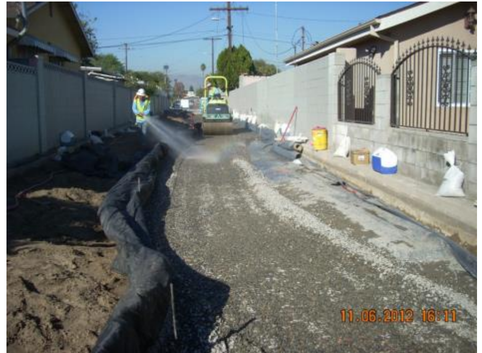
Construction of bio-swale, infiltration trench, and pathway continued.
