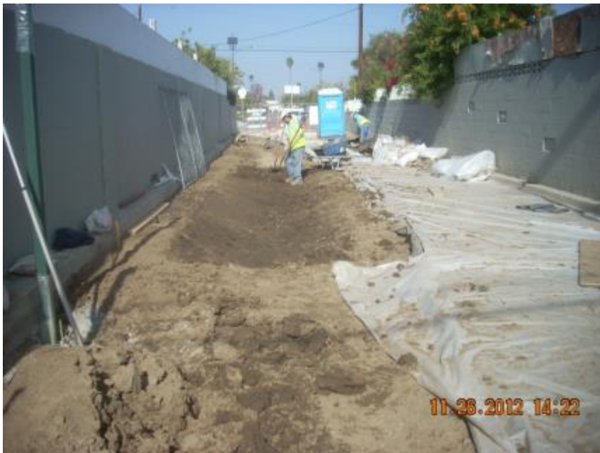
Fine grading for bio-swale
