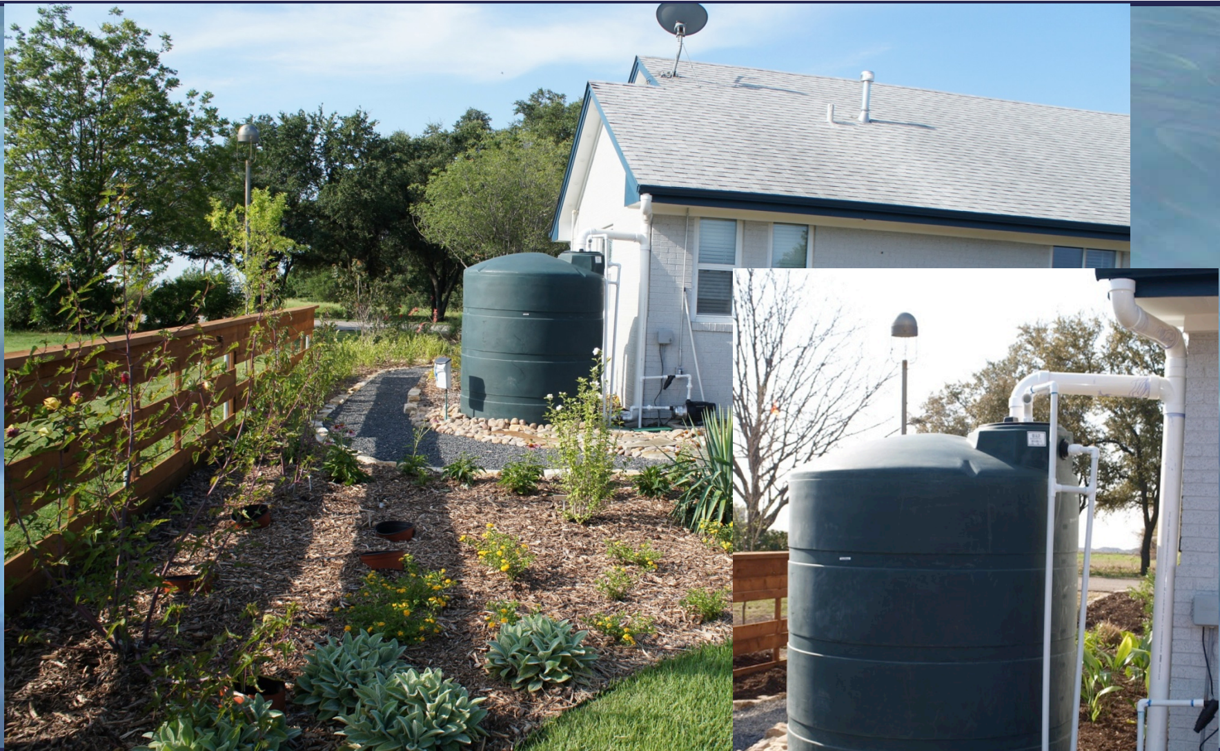
Irrigation Supplied By Rainwater Cistern
