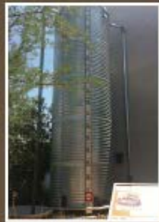
3,800 gallon above-ground cistern
