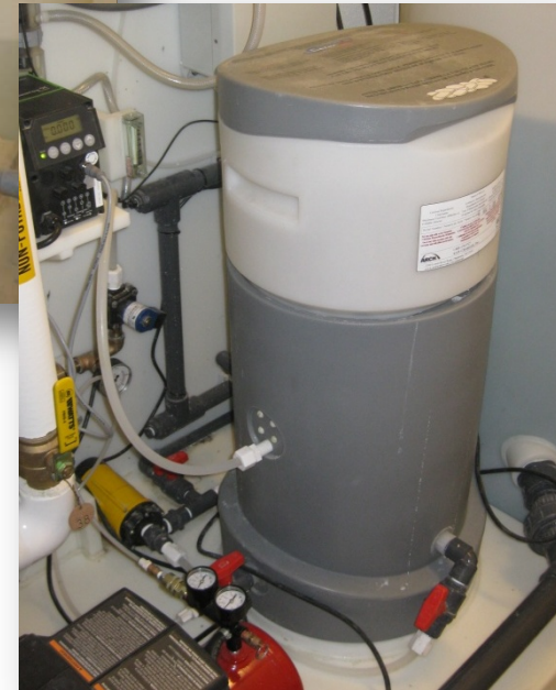
Chlorine Dosing Systems
