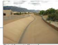
Tinted Concrete Channel
