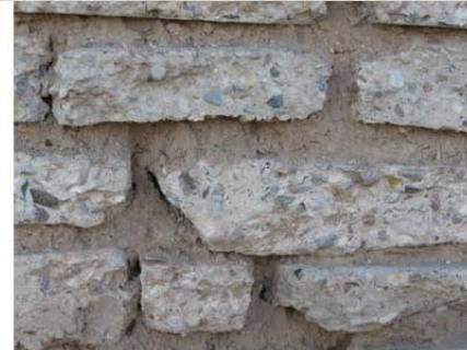
RECYCLED CONCRETE WALL
