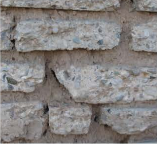
RECYCLED CONCRETE WALL
