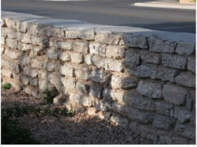
RECYCLED CONCRETE WALL
