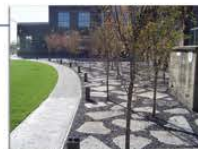
Recycled Concrete & Asphalt Paving
