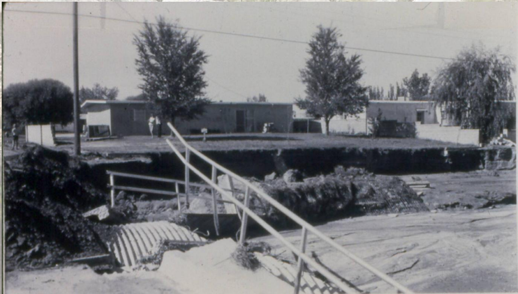
Downstream side of Hahn Arroyo crossing at Washington NE. Wall extended entire length of this yard at Delamor & Washington. (8-13-63)
