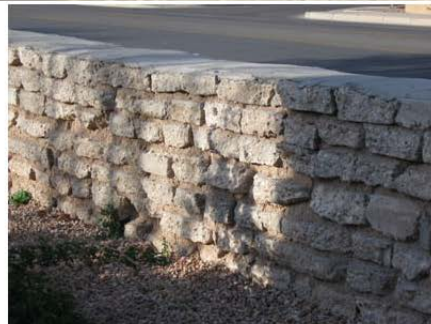
RECYCLED CONCRETE WALL
