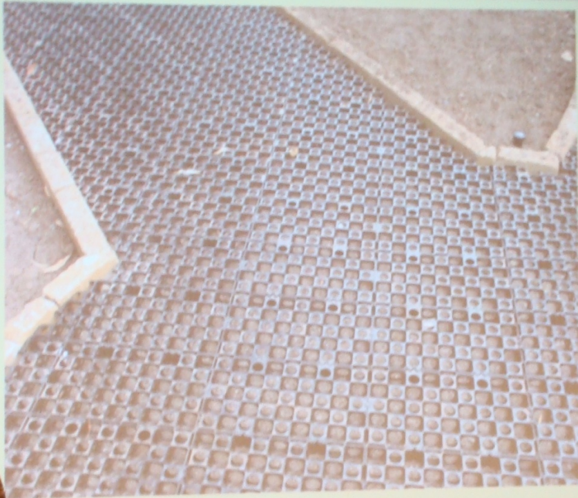
Gravelpave Grid Laid on Sandy Base
