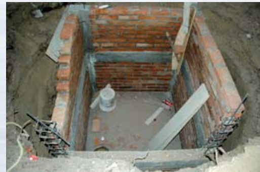
Aljibes Underground water cisterns
