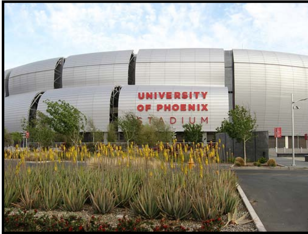
University of Phoenix Stadium
