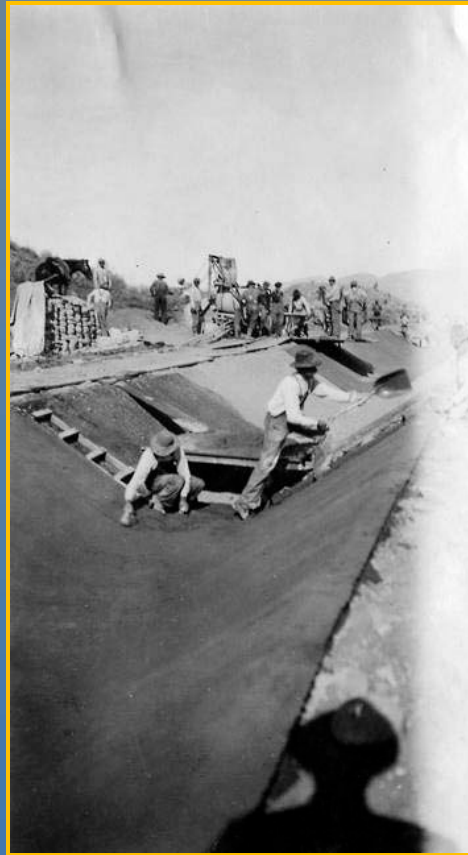
Concrete canal lining project, 1913
