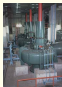
⑤給水所 (本郷給水所配水ポンプ) Water Supplying Station (Hongo Water Supplying Station Distribution Pumps)
