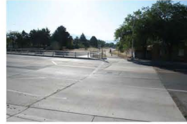
Unsafe Pedestrian Crossing
