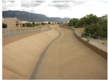
Improved, Tinted Concrete Channel
