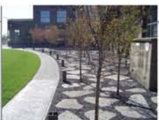
Recycled Concrete & Asphalt Paving
