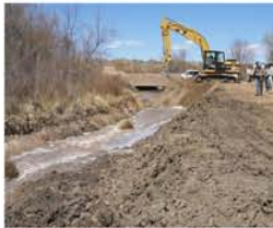
Wetland Restoration: Excavating Channel
