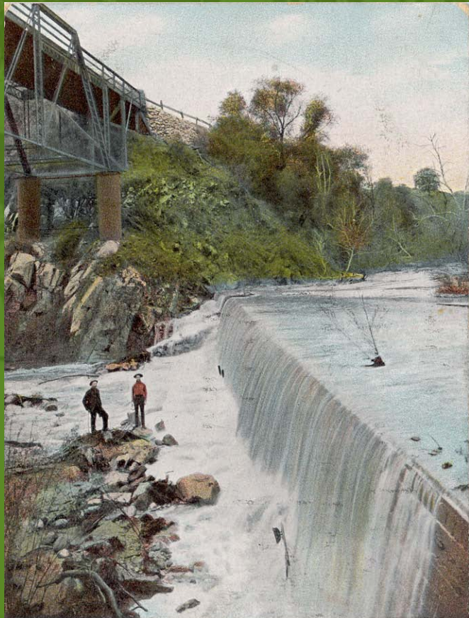
Devil's Gate, Water Supply of Pasadena, Cal.
