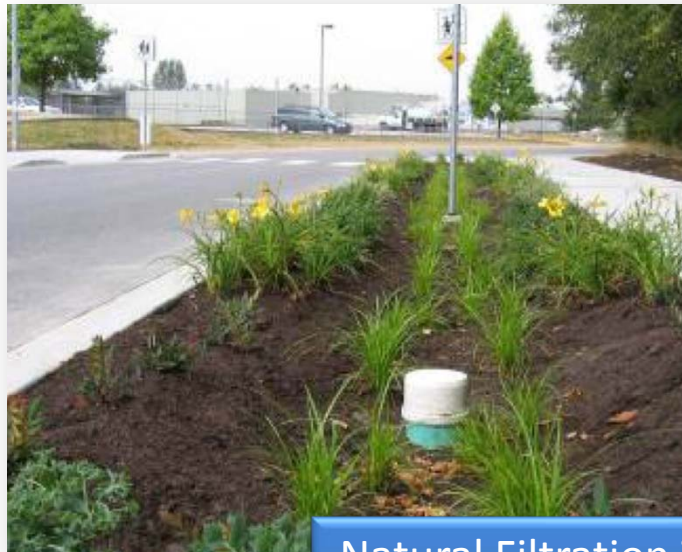
Natural Filtration Through Vegetated Swale
