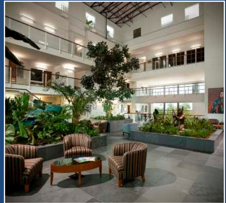
1,200 gpd Living Machine and AC condensate harvesting system inside office building
