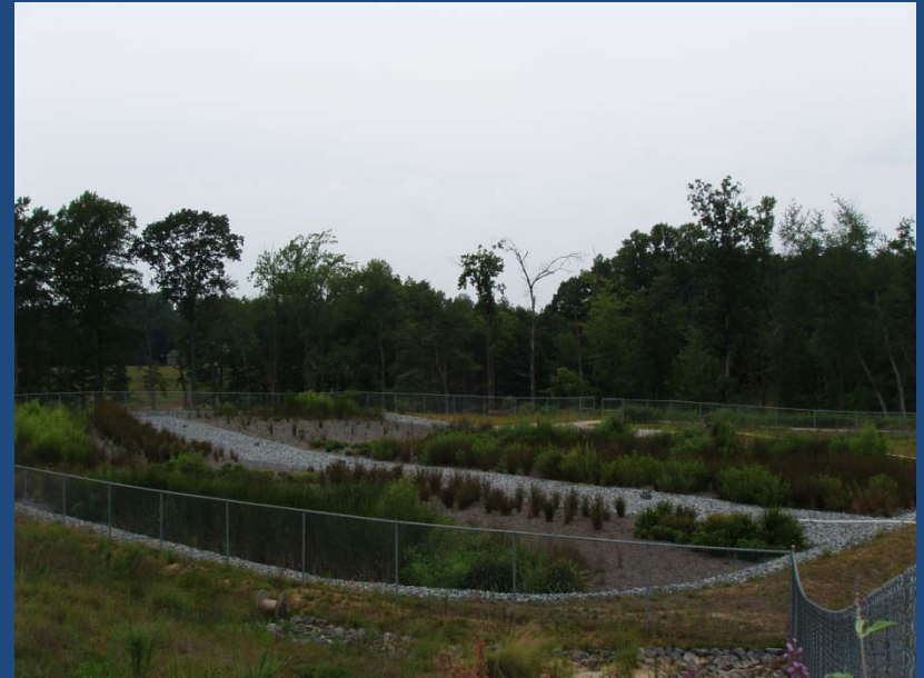
30,000 gpd Living Machine ® system, Southeast USA
