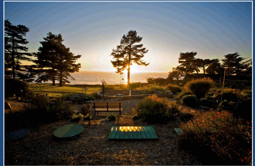
5,000 gpd Living Machine® system, Big Sur, CA
