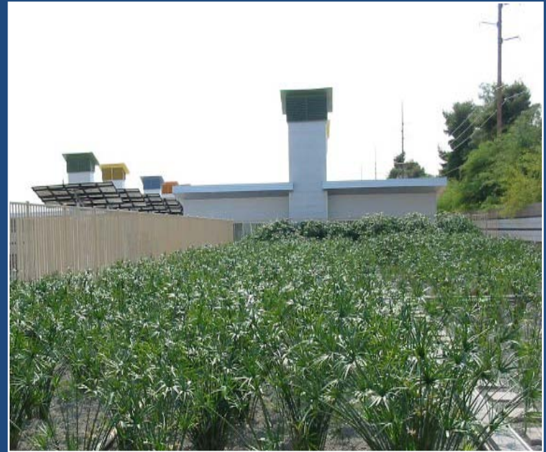
Animal Shelter, Southwest USA, 30,000 gpd
