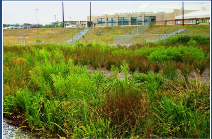
25,000 gpd Tidal Flow® Wetland at a School in Southern USA
