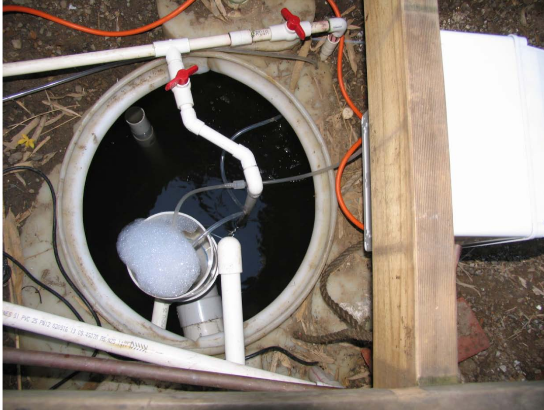
Treatment and storage tank 264 gal.
