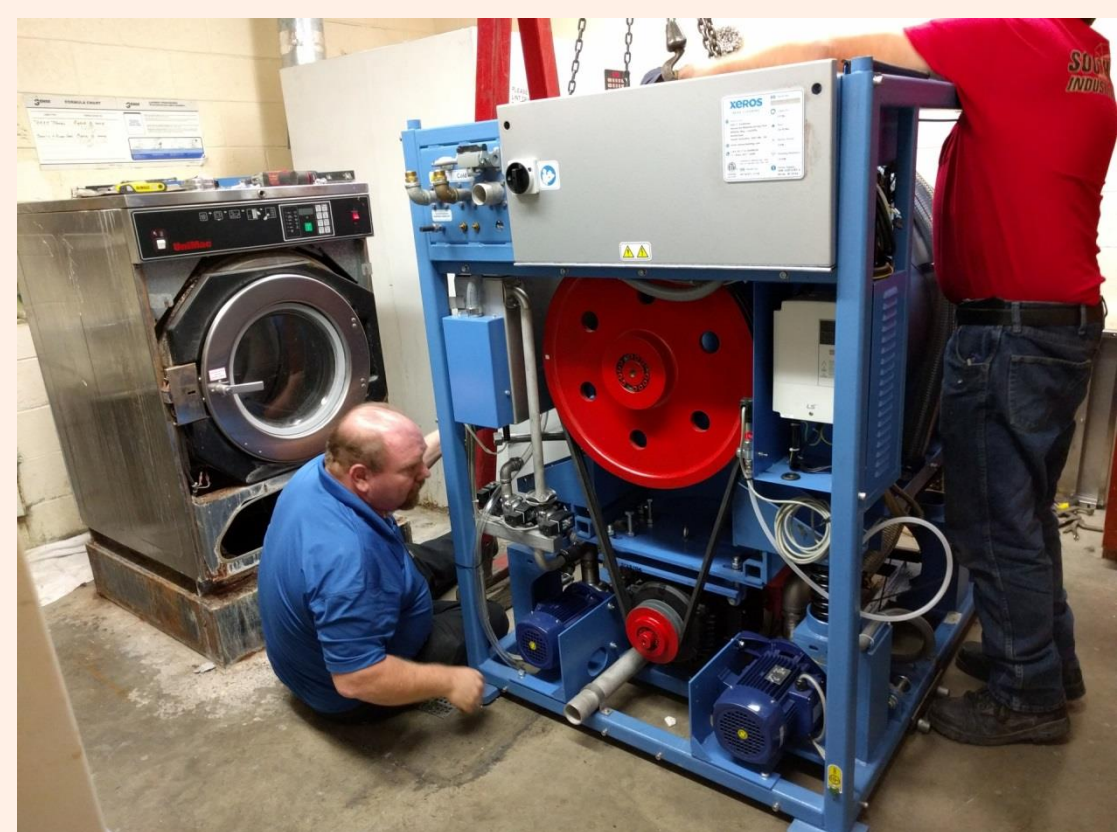
35-lb. Xeros machine installation
