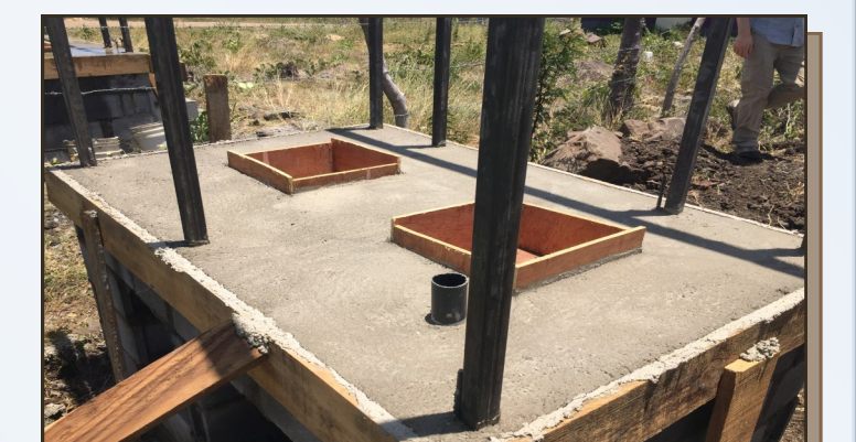
Poured-in-place slab, Photo credit: Andre Ibarra
