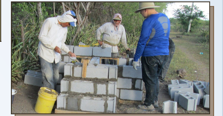
Pit walls, Photo credit: Victor Oliva
