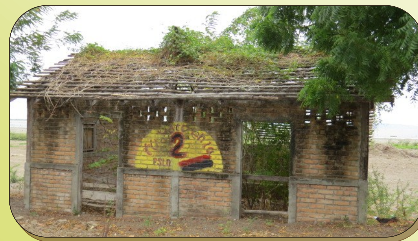
Flooded home near Lake Managua. Photo credit: Katie Hanten
