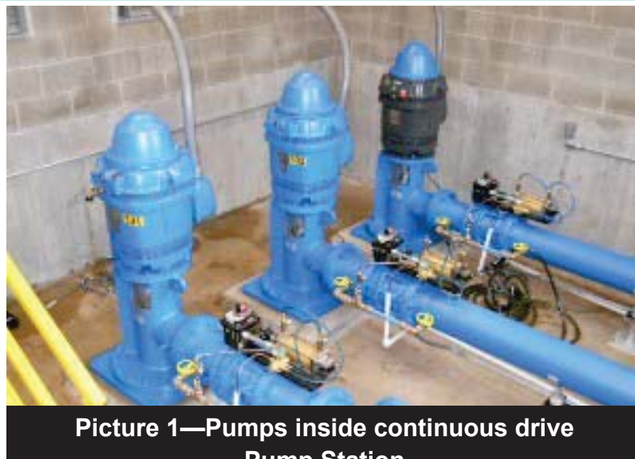
Picture 1—Pumps inside continuous drive Pump Station
