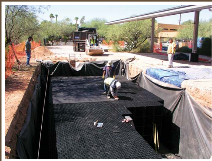
30,000 gallon underground cistern
