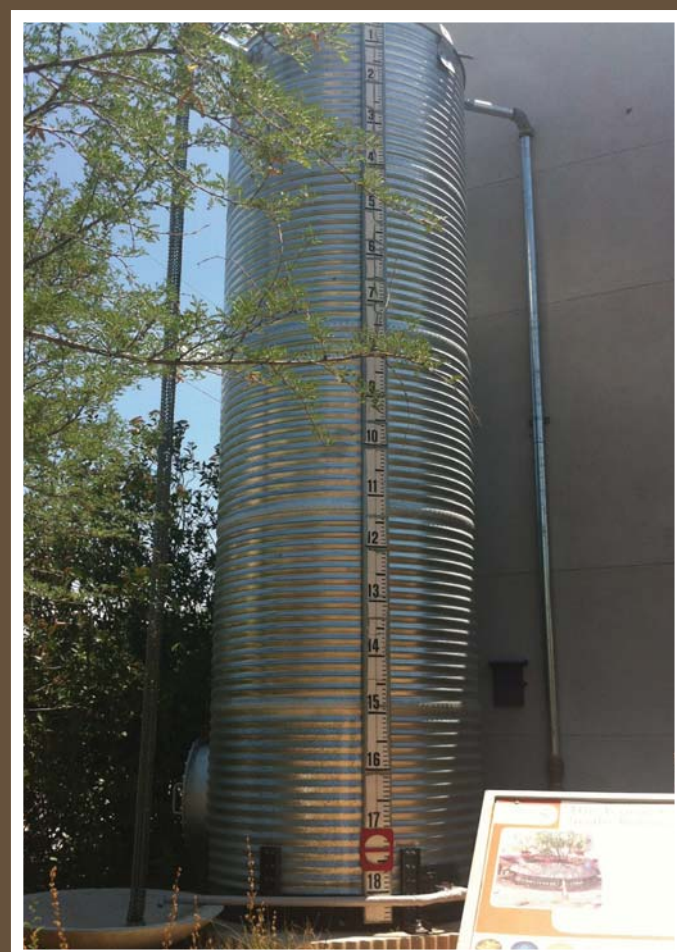
3,800 gallon above-ground cistern
