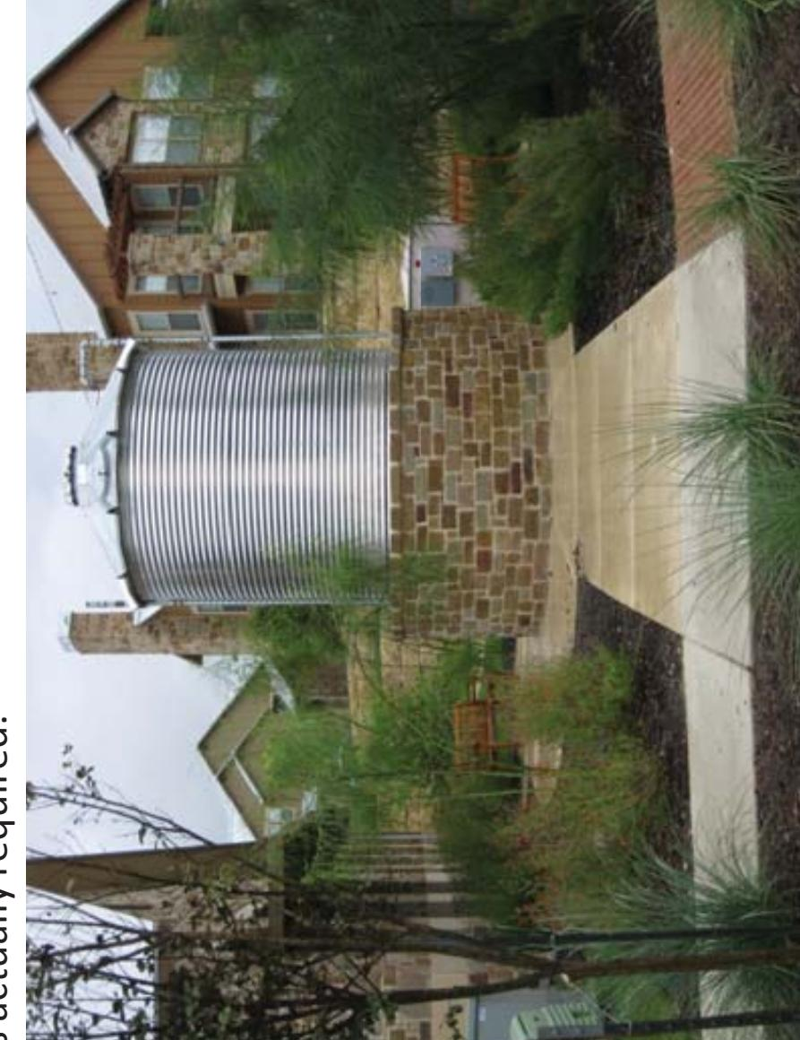
The term "green biling" has been used to refer to projects where the storage is so small that savings from the system will be insignificant. This attractive 10,000 gallon tank is prominently displayed at an apartment complex, but connected to a system that draws over 50,000 gallons for one irrigation cycle.
