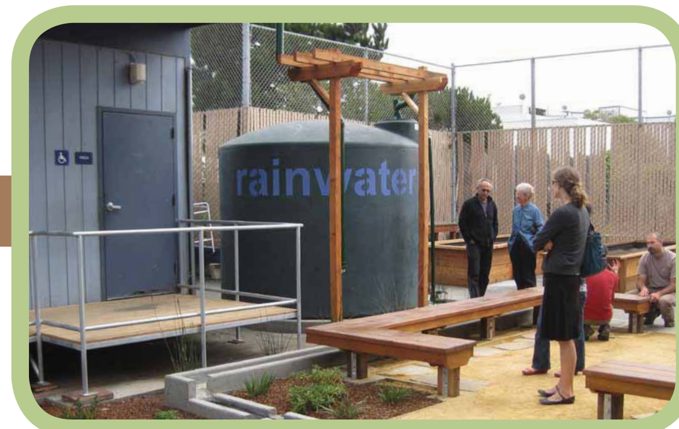
Cisterns range in size from 620 to 5500 gallons. Rainwater can be used on edibles or native plants.
