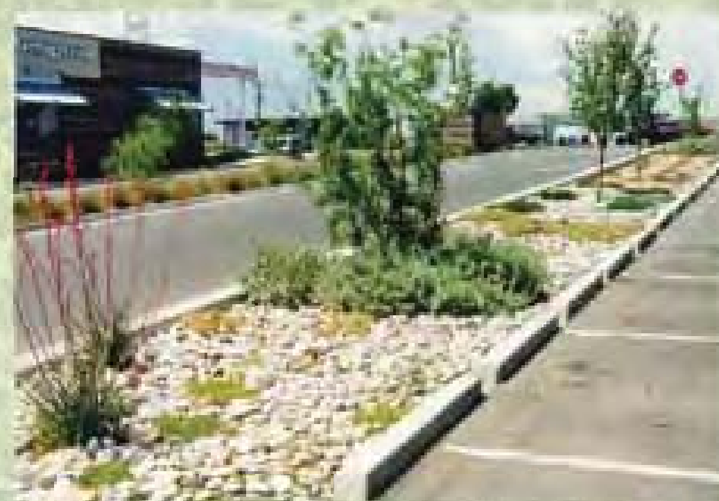
Water Harvesting Median in Shopping Center
