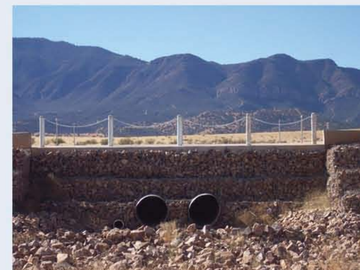
Water retention basins aid in recharge.
